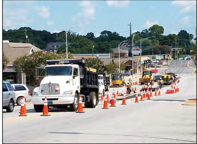
Sewer Main Replacement Project on College Street
