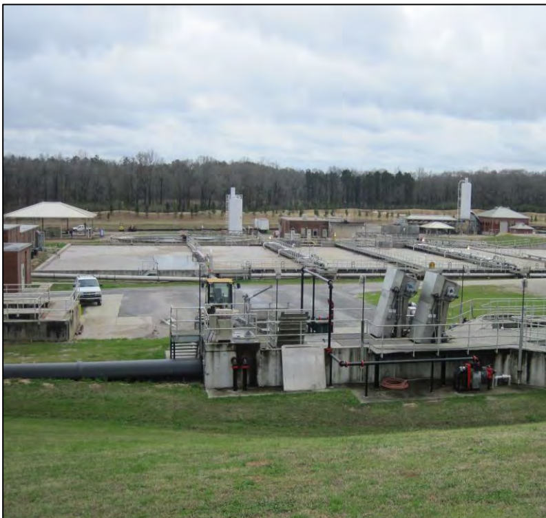
H.C. Morgan Water Pollution Control Facility
