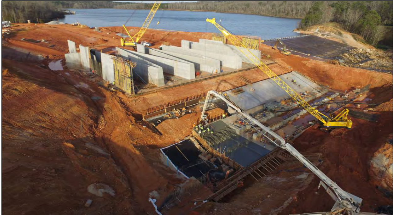
Lake Ogletree Spillway Construction
