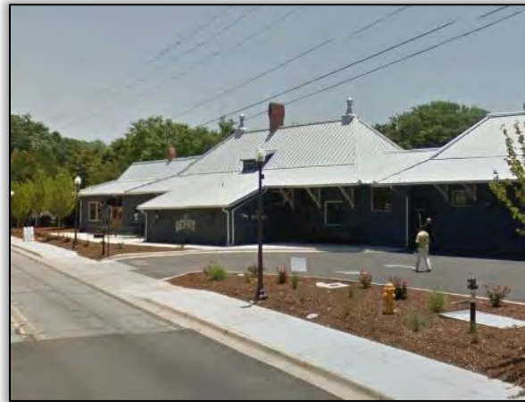
Auburn Depot, 120 Mitcham Avenue – 2016
