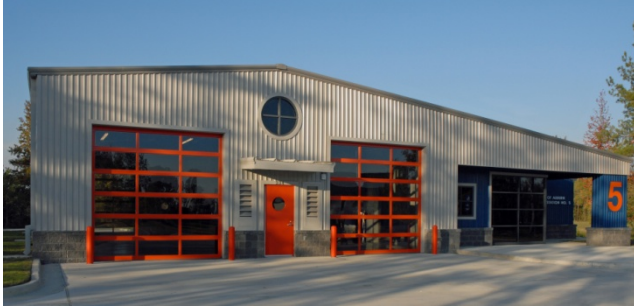
Fire Station No. 5 opened in November 2007.
