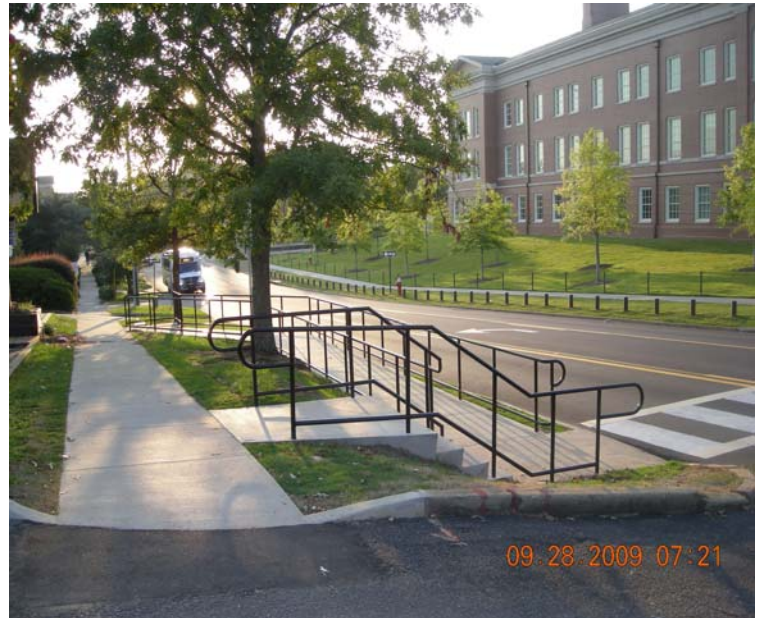
West Magnolia Avenue Pedestrian Improvements and Road Reconstruction
